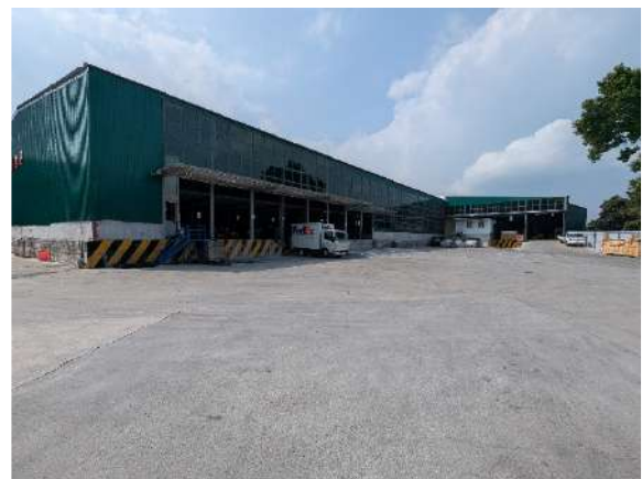
Photo No. 2 – Hard paved within the Application Site (2 of 2)
