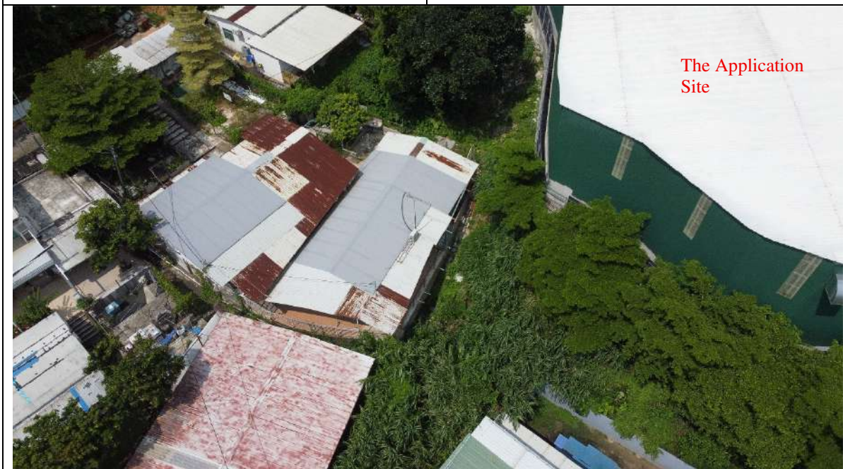
Photo No. 5 – View along the eastern boundary of the Application Site
