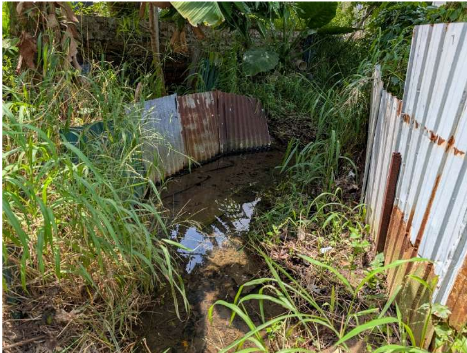
Photo No. 15 – Close up view at the existing watercourse at the further downstream (2 of 2)
