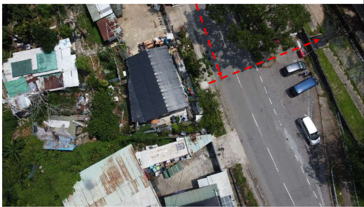
Photo No. 20 – Existing underground drainage discharging into the existing 22m wide trapezoidal channel beside Kam Ho Road
